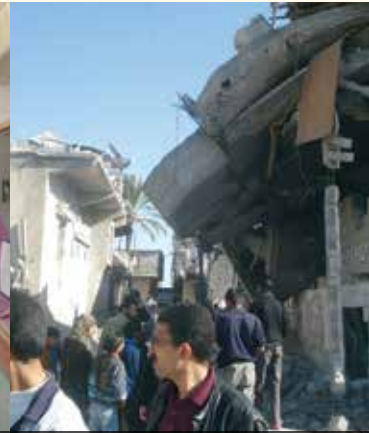
A destroyed building in Gaza during the 2008-09 Gaza war.
