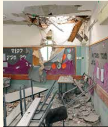
Hamas rocket damage to a classroom during the 2008-09 Gaza war.
